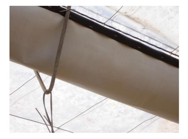
The VRG is offered in black & white(the white color is positioned towards the inside of the to the greenhouse, to reflect the light ) or in black only.
